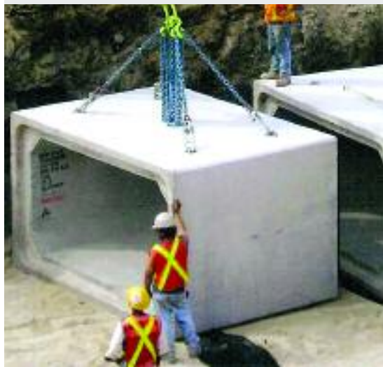
Just-in-time delivery and standard box sizes accommodated installation.
